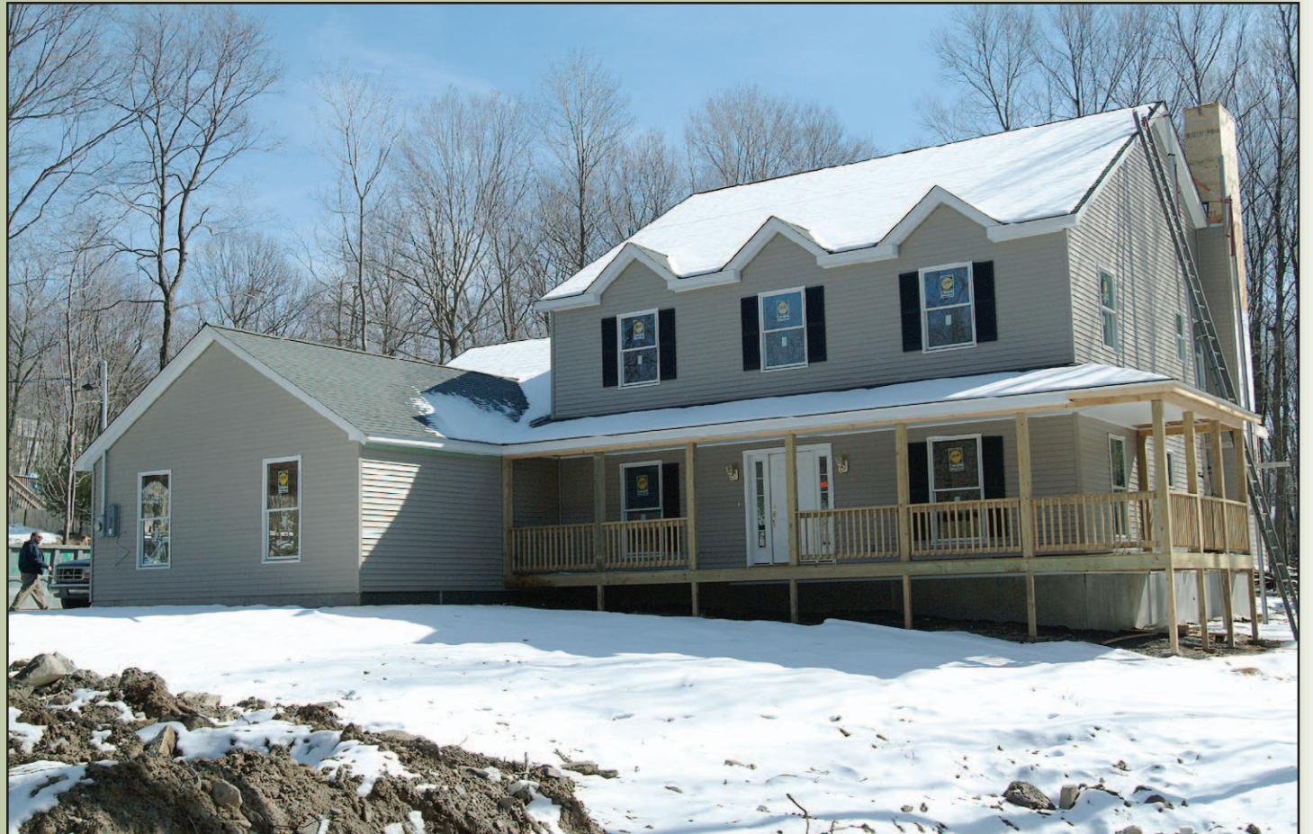
This farmhouse-colonial modular home was delivered to its site in seven sections.
